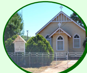
Anglican Church Wattle Street, Tullibigeal
