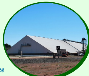
Grain Handling Facility Burgooney Road, Tullibigeal
